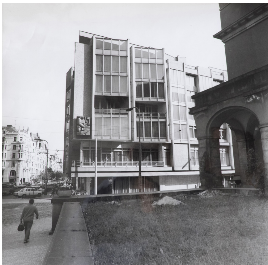
Figure 16 The new IUS building, 1974. Source: Courtesy of Radan Hubička and Radim Hubička.
